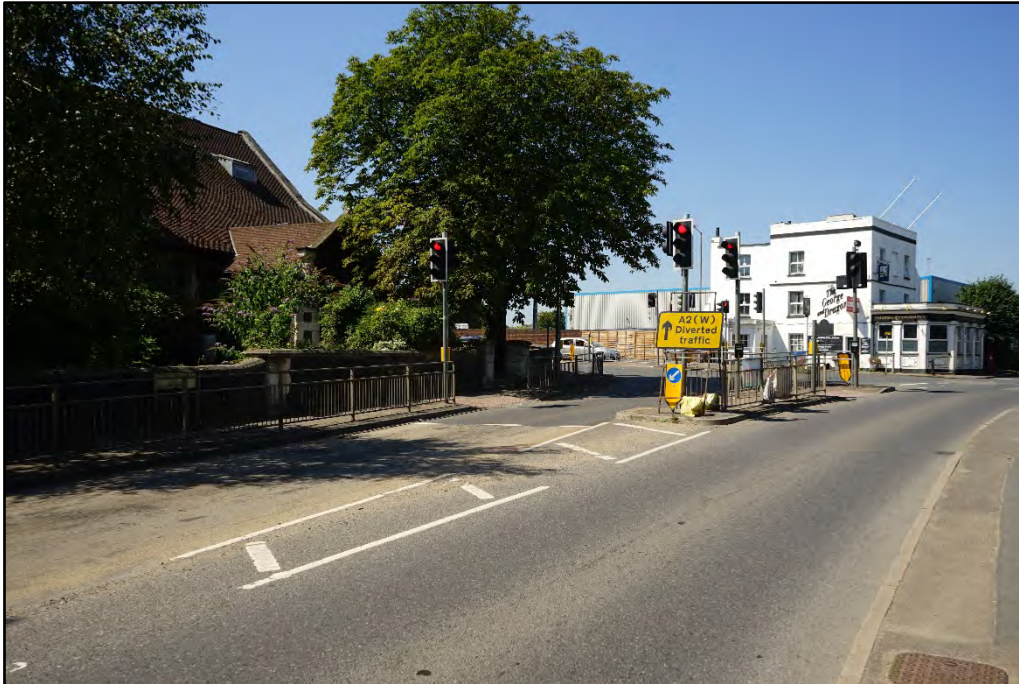
Plate 26: View of All Saints Church in conjunction with the George and Dragon public house, facing west-southwest from London Road
