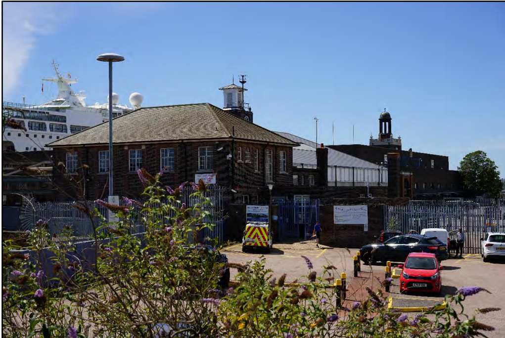
Plate 1: Overview of the Riverside Station's north and east elevations, viewed from the east – note detrimental palisade fencing
