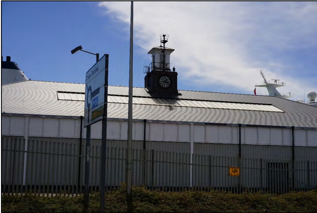
Plate 3: Much altered north elevation of the former station building
