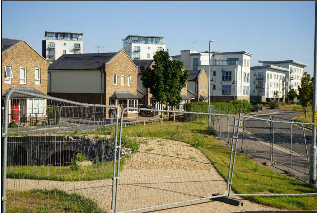
Plate 9: View north along the Kent Project Site's western boundary, with the Listed Garden Bridge, Ingress Abbey on the left
