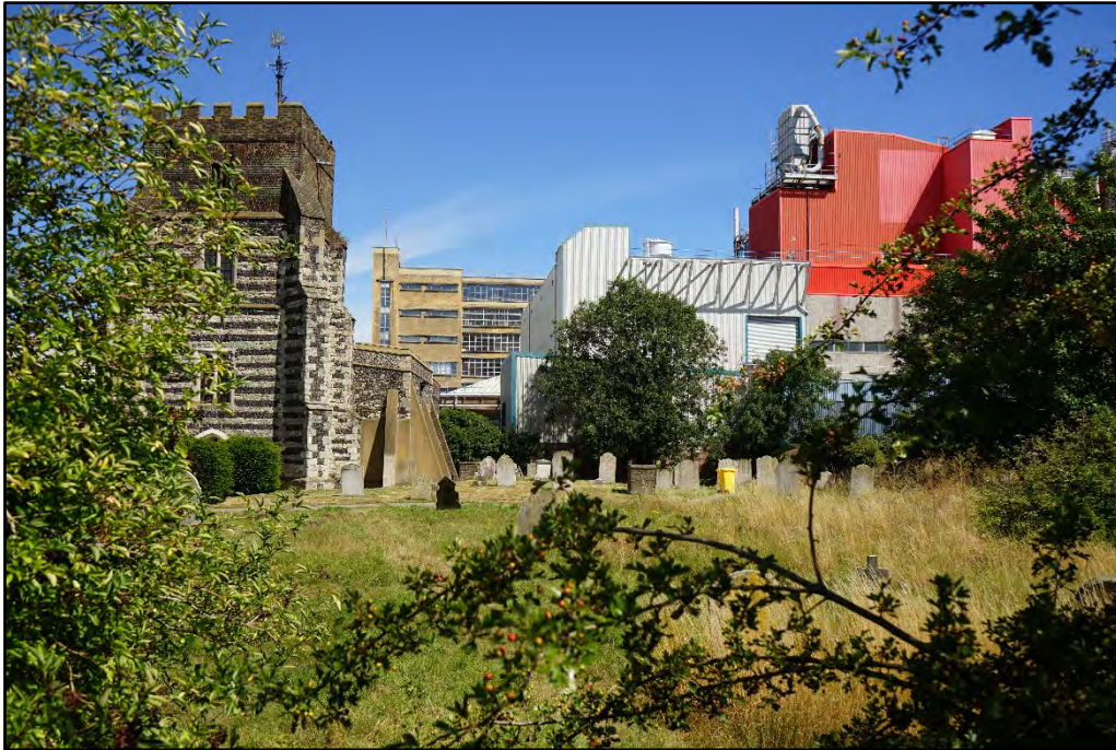
Plate 34: View to the west elevation of the Church of St Clement with factory building just beyond
