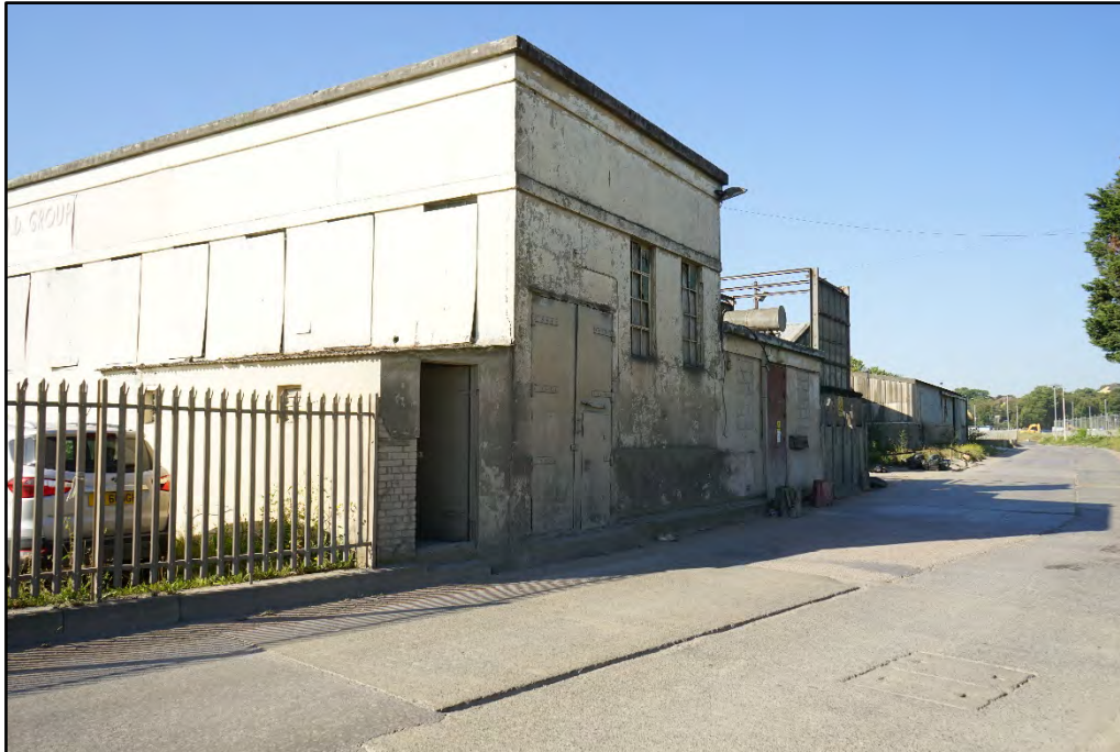
Plate 40: Former Portland Cement Works sub-station (left) with the warehouse (back right), facing southwest along Manor Way
