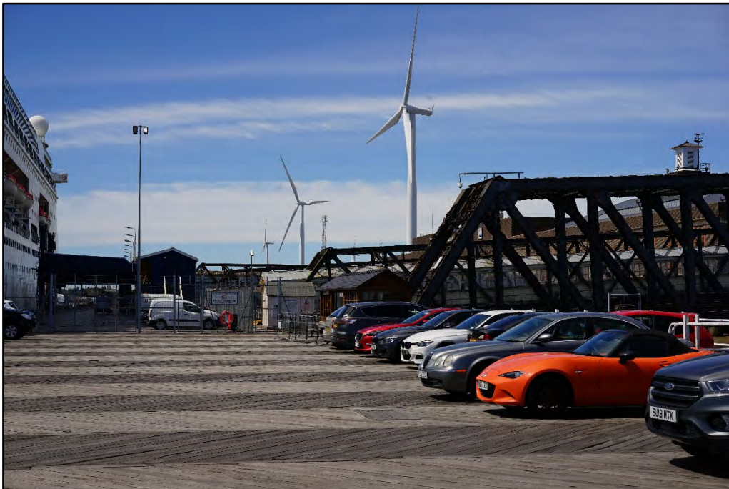
Plate 2: View west along the landing stage of the Riverside Station from its eastern end
